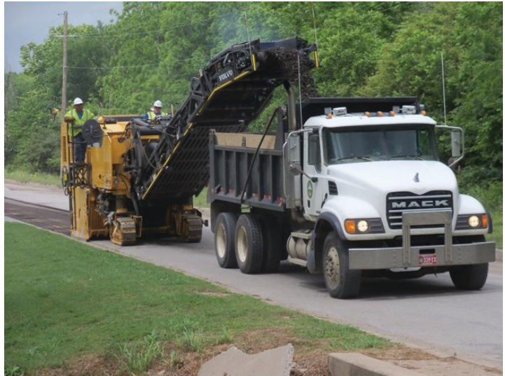
The Muscogee (Creek) Nation purchased a Volvo MT2000 milling machine to maintain roads in their Jurisdiction Area.
